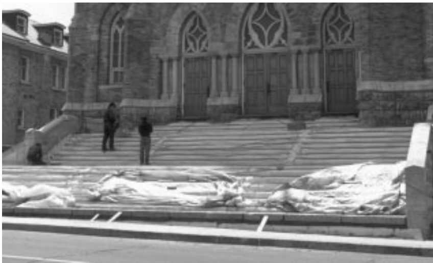
Fig. 1.2 Installation of RAUPEX SIM system on church steps
