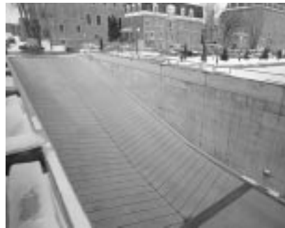
Fig. 1.6 Completed parking garage ramp
