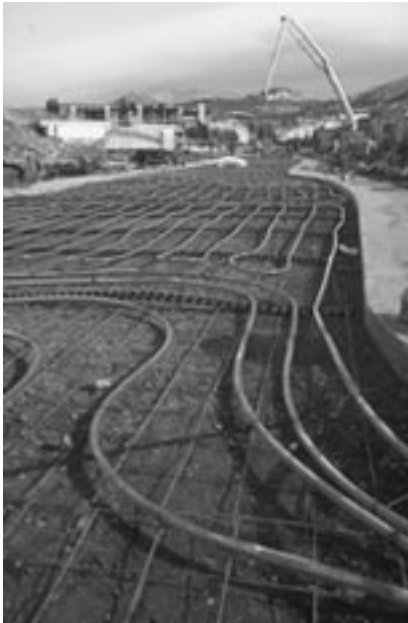
Fig. 4.1 SIM system installation beneath roadway
