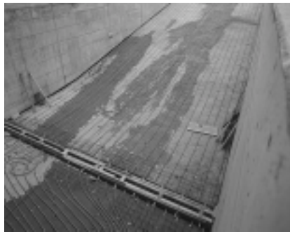
Fig. 1.5 Parking garage ramp RAUPEX B installation
