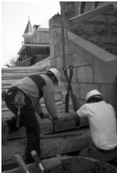
Fig. 3.2 SIM church step installation
