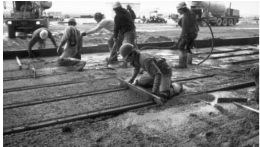
Fig. 3.3 Concrete installation over SIM system
