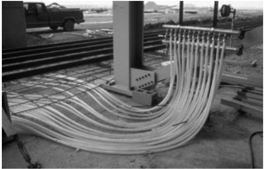
Fig. 2.3 SIM distribution manifold
